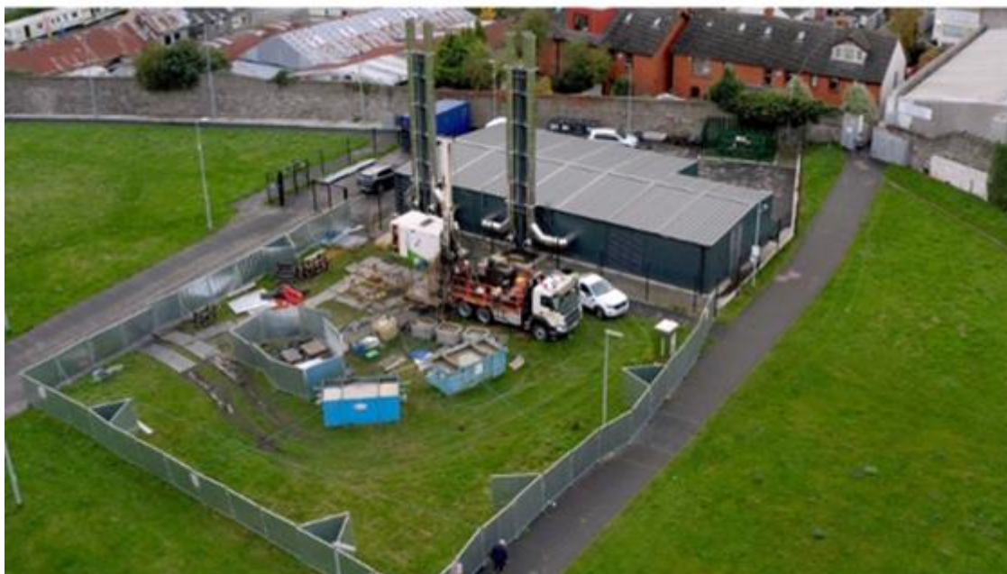
Figure 23 – Borehole at TUD
